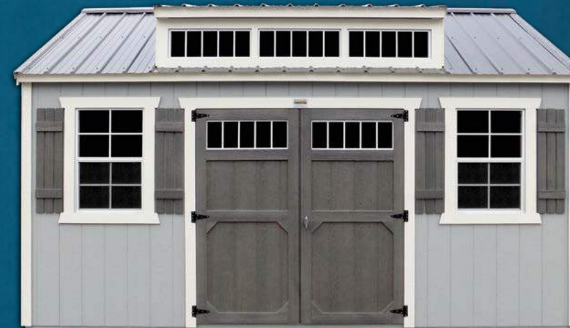
GAP GRAY PAINT, NAVAJO TRIM PAINT & DRIFTWOOD URETHANE ON SHUTTERS & DOORS ON LP SMART PANEL SIDING
